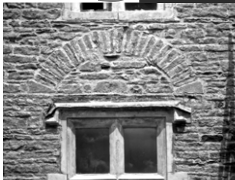
Restoration of Lodge Farm Mangotsfield Steve Rendell B.A(Hons), B.Arch (Nottm)
